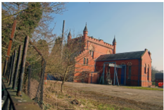
The Bratch Pumphouse is about 1/4 mile from Wombourne Station
