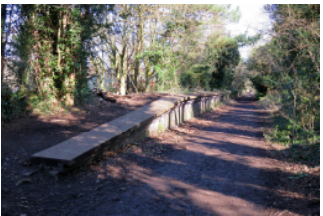
The platform face at Compton Halt is still intact
