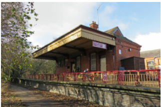
Tettenhall Station is now home to Cupcake Lane tearoom
