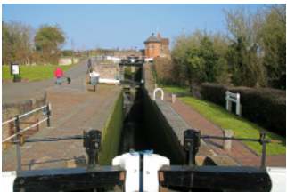
The Bratch Locks are just past the Pumphouse
