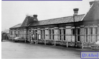
Stourbridge Town Station Building
