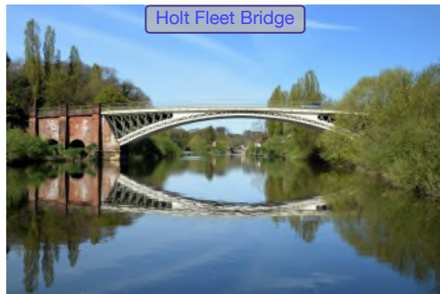
Holt Fleet Bridge
